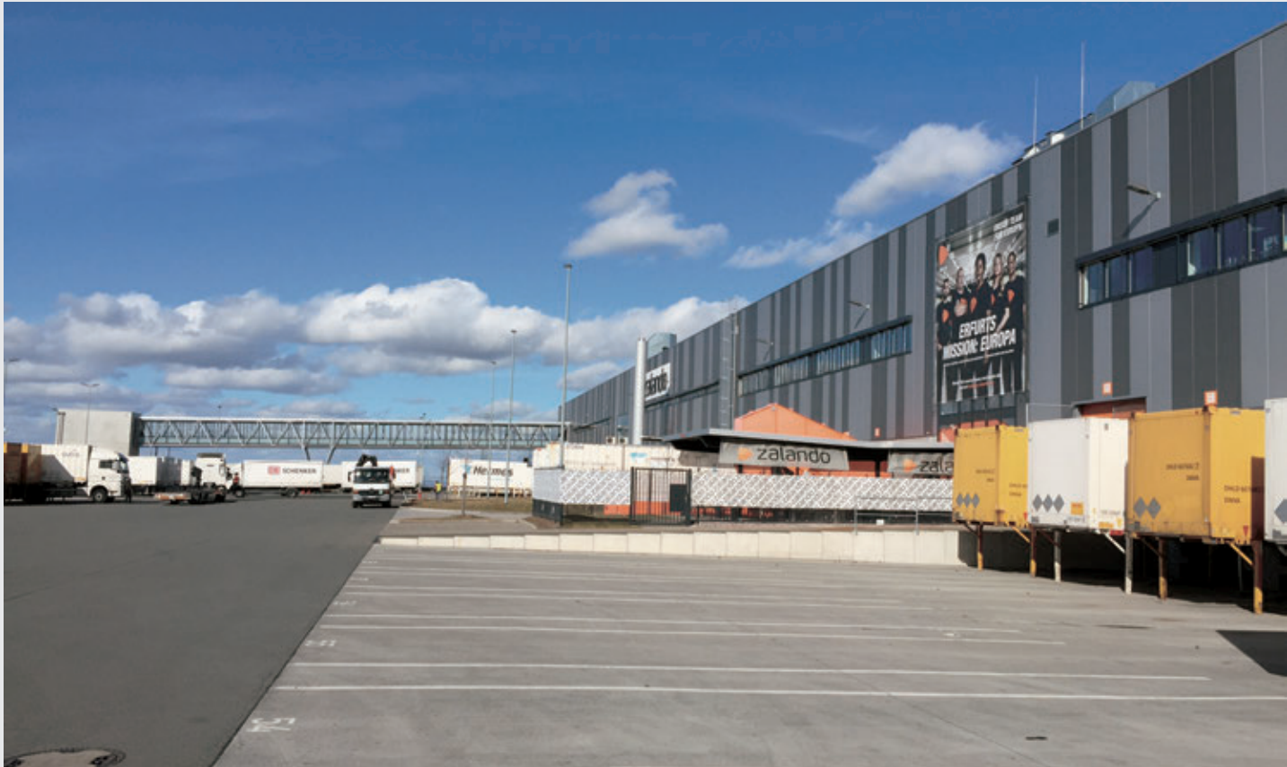
Zalando Distribution Warehouse, Erfurt, Jerman
