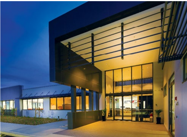
133 LENORE DRIVE, ERSKINE PARK, SYDNEY, AUSTRALIA (LOGISTIK)
